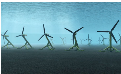
Underwater 10 megawatt tidal stream project in the Sound of Islay between the Hebridean islands of Islay and Jura. (Credit: ScottishPower Renewables)
