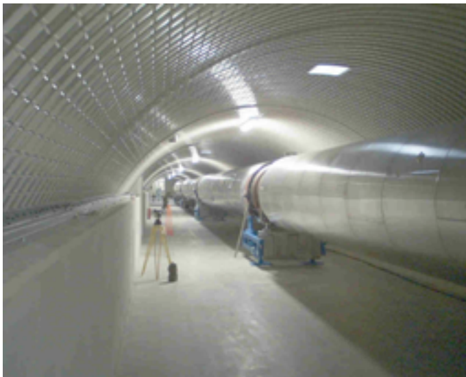
Figure 1 - The Virgo North arm Vacuum pipe; 3 km long, 1.2 m diameter.
