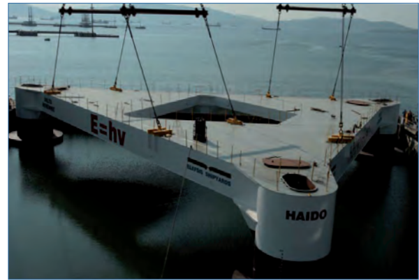
View of the astroparticle-physics dedicated boat under construction in Pylos (Credit: NESTOR collaboration).
